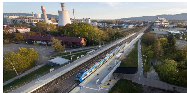
Reconstruction of railway line No. 139 Intop Warszawa Sp. z o.o.
