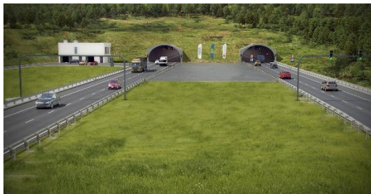
Expressway S3 - task 3 PORR S.A.
