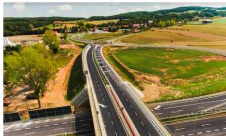
Expressway S3 - task 2 Mota-Engil Central Europe S.A.
