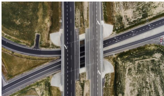
Expressway S3 - task 4 Mota-Engil Central Europe S.A.
