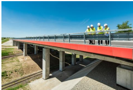
Nysa Bypass - National Roads Mota-Engil Central Europe S.A.
