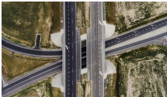
Expressway S3 - task 4 Mota-Engil Central Europe S.A.
