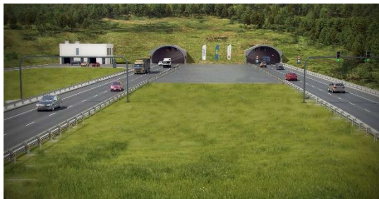
Expressway S3 - task 3 PORR S.A.
