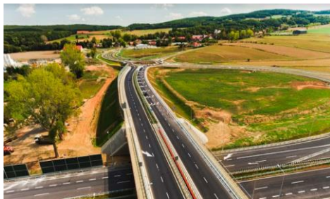
Expressway S3 - task 2 Mota-Engil Central Europe S.A.
