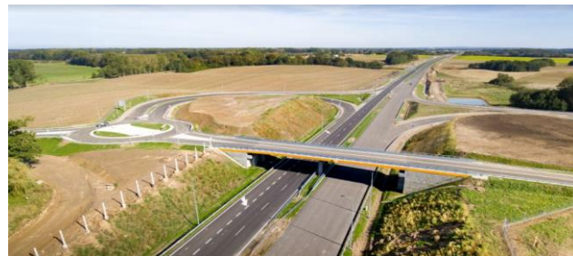
Expressway S6 Strabag Sp. z o.o.
